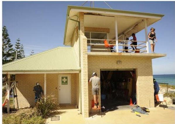
Swanny at work - volunteer patrol tower maintenance works
